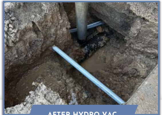
AFTER HYDRO VAC
