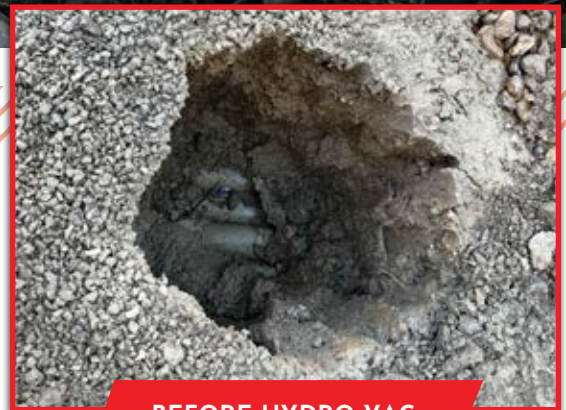
BEFORE HYDRO VAC
